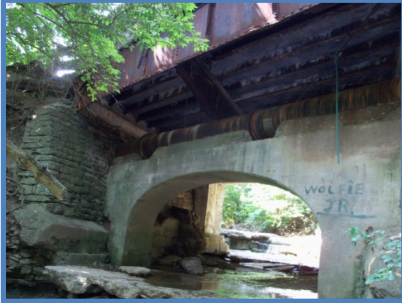
North Side of Bridge Looking South, Utility Line on Arch
