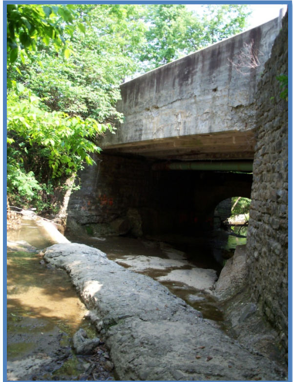
North Side of Bridge Showing Utility, Crack and I-Beam Section Loss
