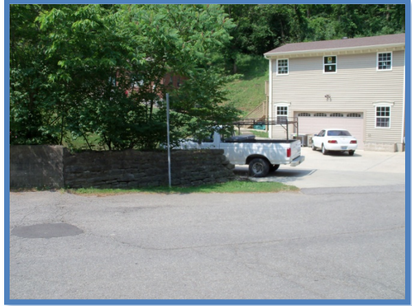
Driveway on South/East Side of the Bridge
