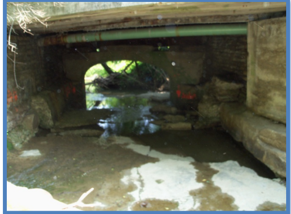
From South (Downstream Side) Looking North to Bridge
