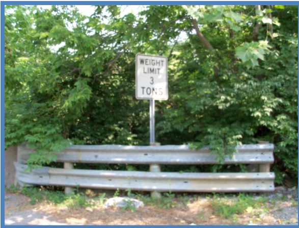
North/East End of Bridge
