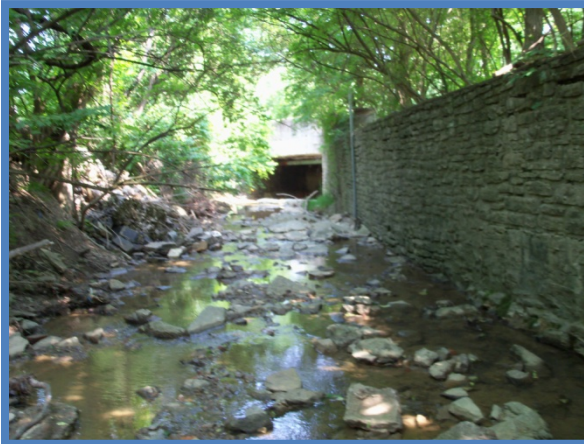
From South (Downstream) Side Looking North to Bridge
