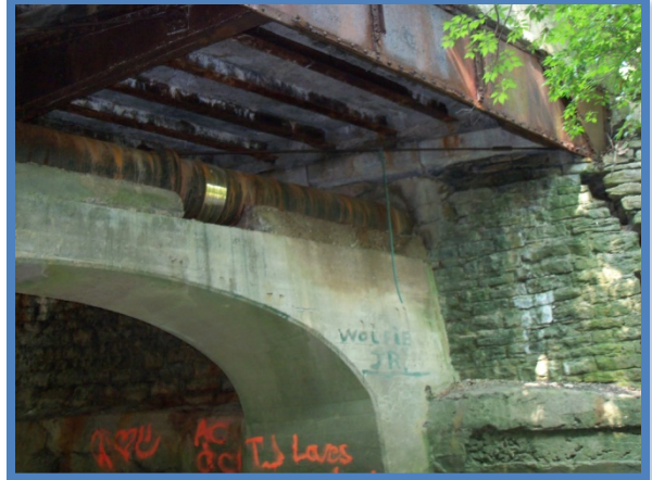
North Side of Bridge Showing Utility, Crack and I-Beam Section Loss
