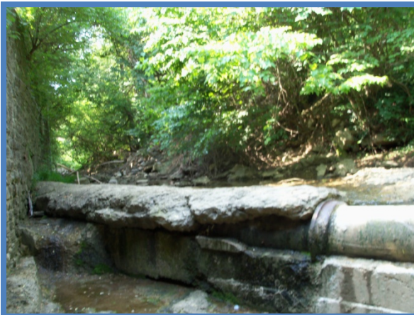
Utility on South Side of Bridge
