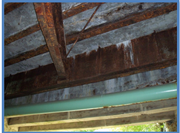
Close-up of Waterline Going Through the Bridge
