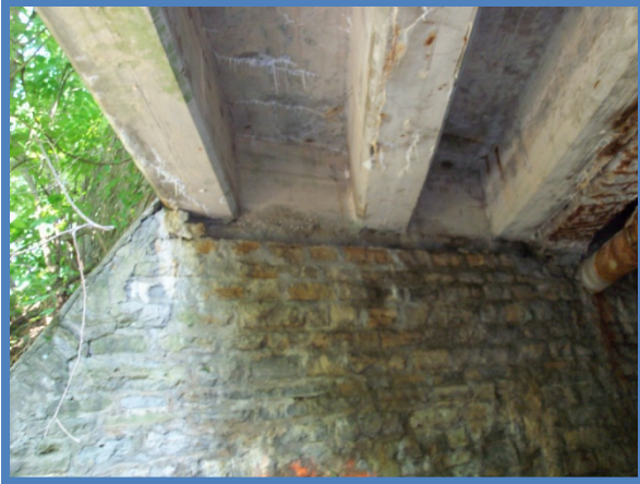
South Side of Bridge, Concrete Tee Beam Portion
