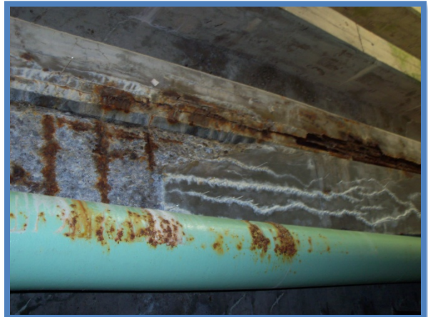
Close-up of Waterline Going Through the Bridge
