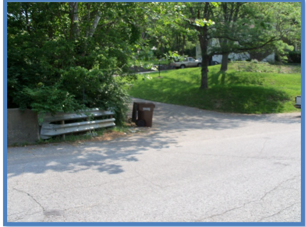
Driveway on North/West Side of Bridge
