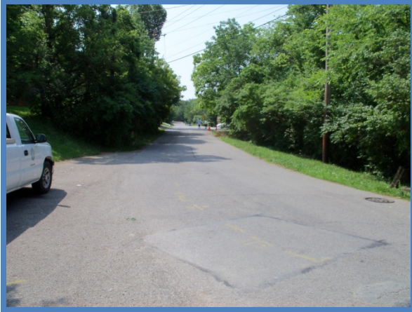
Waterworks Road Looking West
