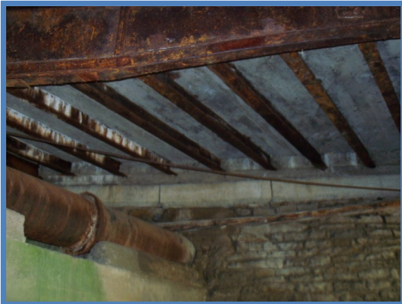
North Side of Bridge, Steel Girder Floorbeam System
